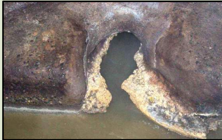
FOG Accumulated in a Manhole Channel
