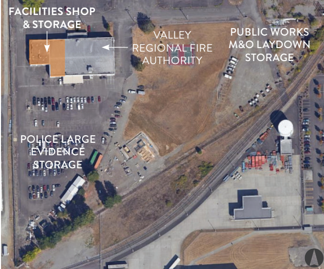
FIGURE 81. FACILITIES SHOP & STORAGE AT GSA PROPERTY
