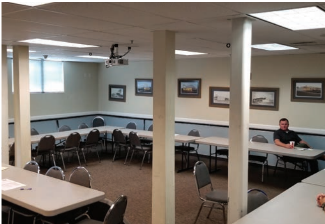
FIGURE 20. POLICE TRAINING ROOM COLUMNS IMPEDE SIGHTLINES FOR CLASSROOM TRAINING
