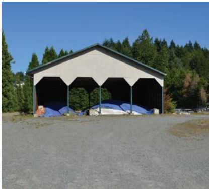
FIGURE 71. COVERED STORAGE AT R STREET PROPERTY
