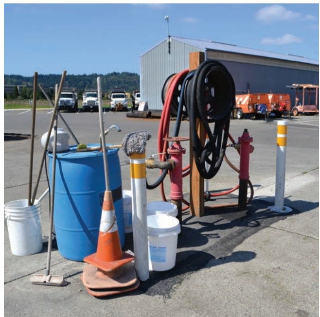
FIGURE 50. EXISTING WASH RACK
