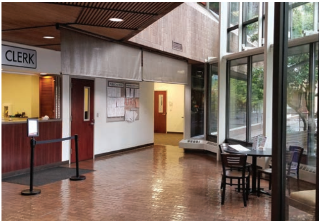
FIGURE 83. THERE ARE PRIVACY AND SECURITY CONCERNS FOR CUSTOMER SERVICE COUNTERS AT CITY HALL
