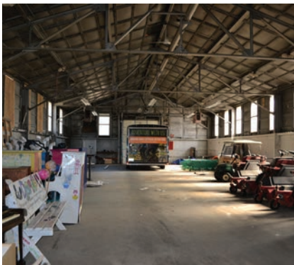
FIGURE 72. RECREATIONAL STORAGE AT R STREET PROPERTY
