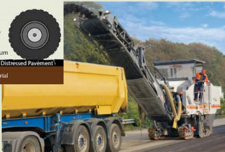
Removal of material
