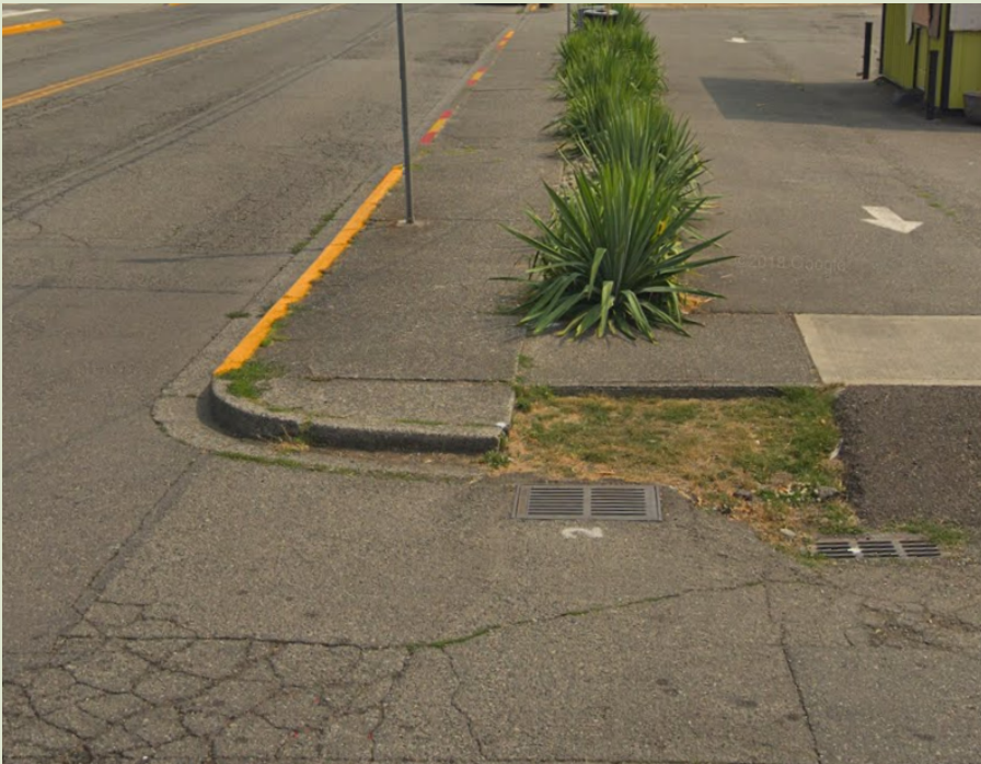
Southeast Corner of B St SE
