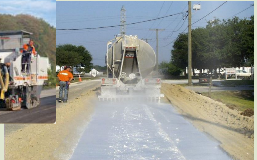
Application of stabilizing Cement
