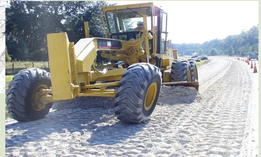
Shape the roadway and compact with a smooth roller
