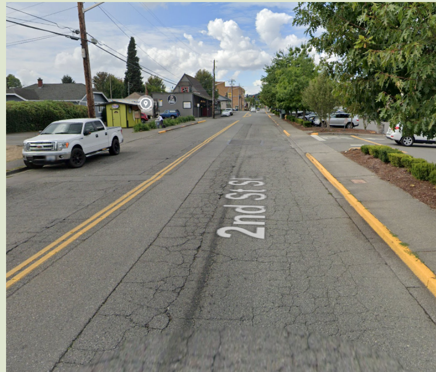
2 nd Street SE – Looking West
