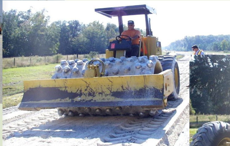
Compact the subgrade
