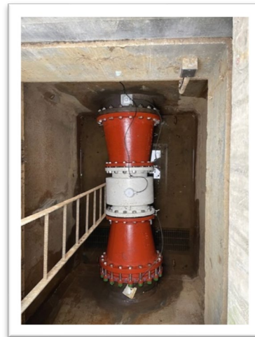
Coal Creek Springs Flowmeters Rehabilitation
