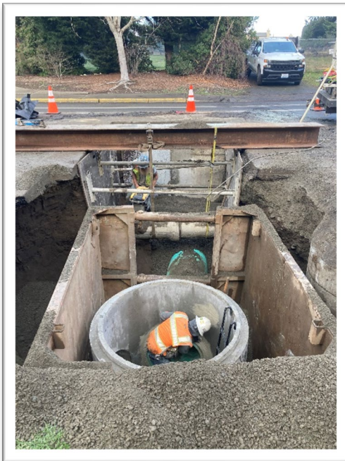
D St SE & 23 rd St SE storm improvements.
