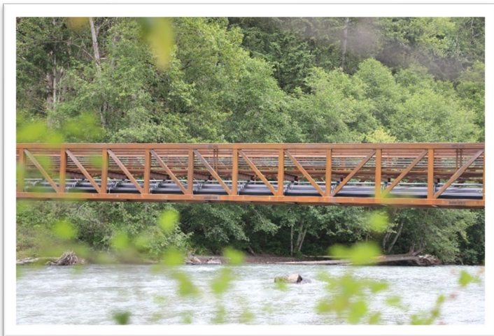
Coal Creek Springs 24-inch Transmission Main
