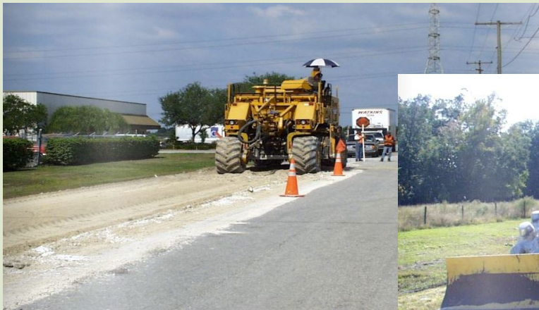
Blend in stabilizing material
