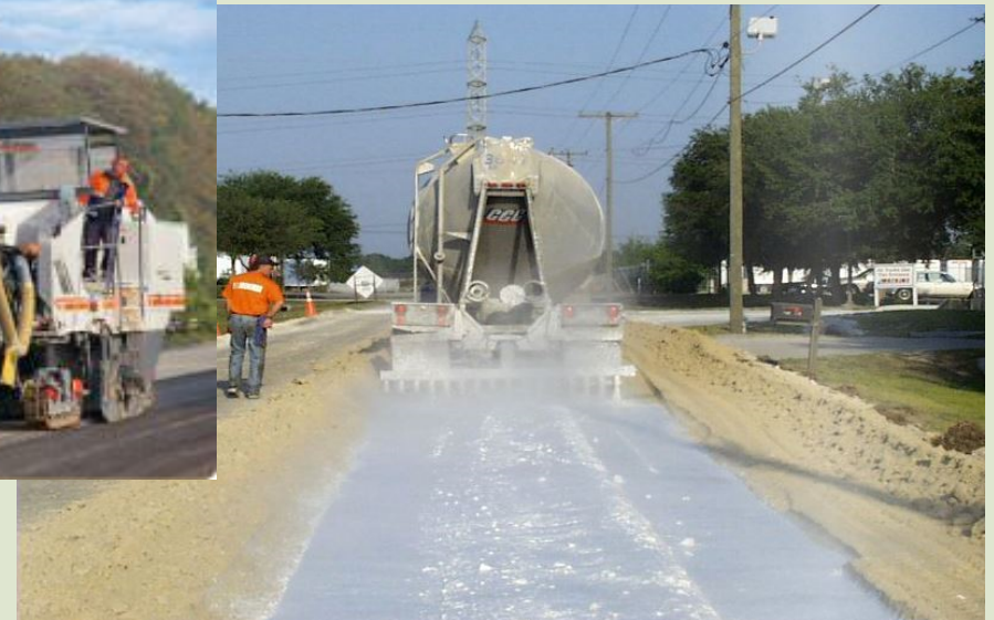
Application of stabilizing Cement
