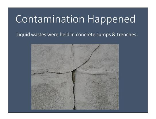
Over time, concrete cracks. The liquids went through the cracks and contaminated the soil under the concrete, and eventually, the groundwater under the soil.
